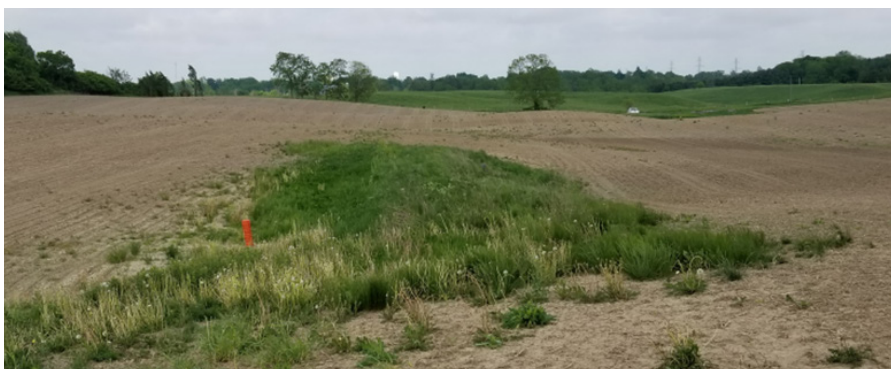
Permanently vegetated narrow-based berm with cropland on either side.
